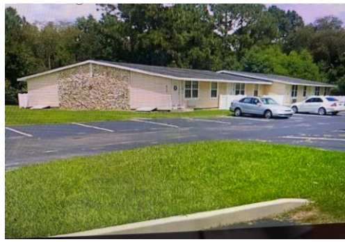
#412D 31 st Avenue SE
